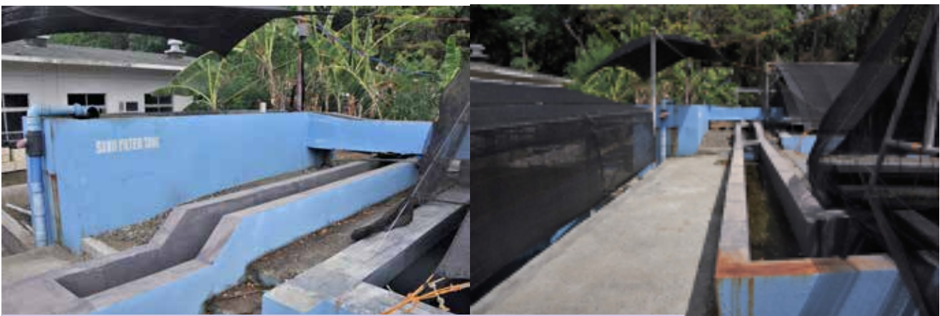
Left: sand filter tank and water supply canal; right: water outlet canal going to the broodstock tank
