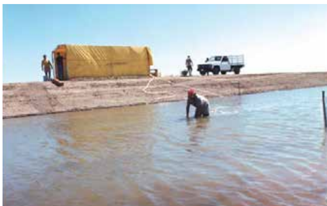
A covered post larvae acclimation station in Peru. Large siphon hoses can be used to drain post larvae directly to ponds from the acclimation tanks.
