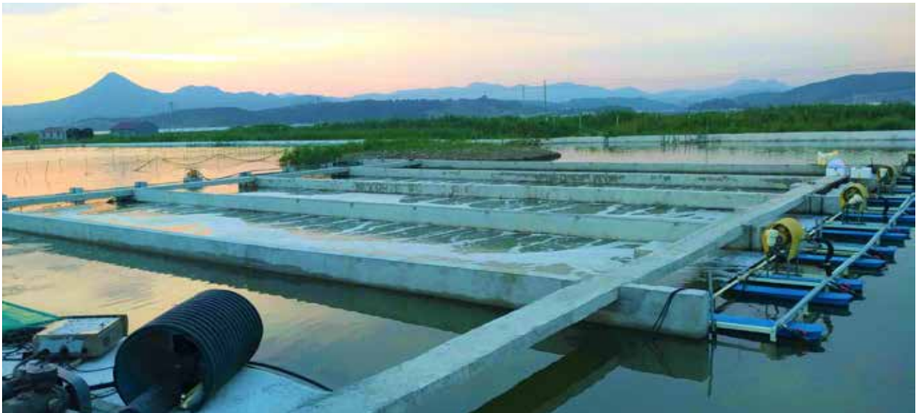
Concrete type Marine IPRS in Ninghai, Zhejiang Province, China
