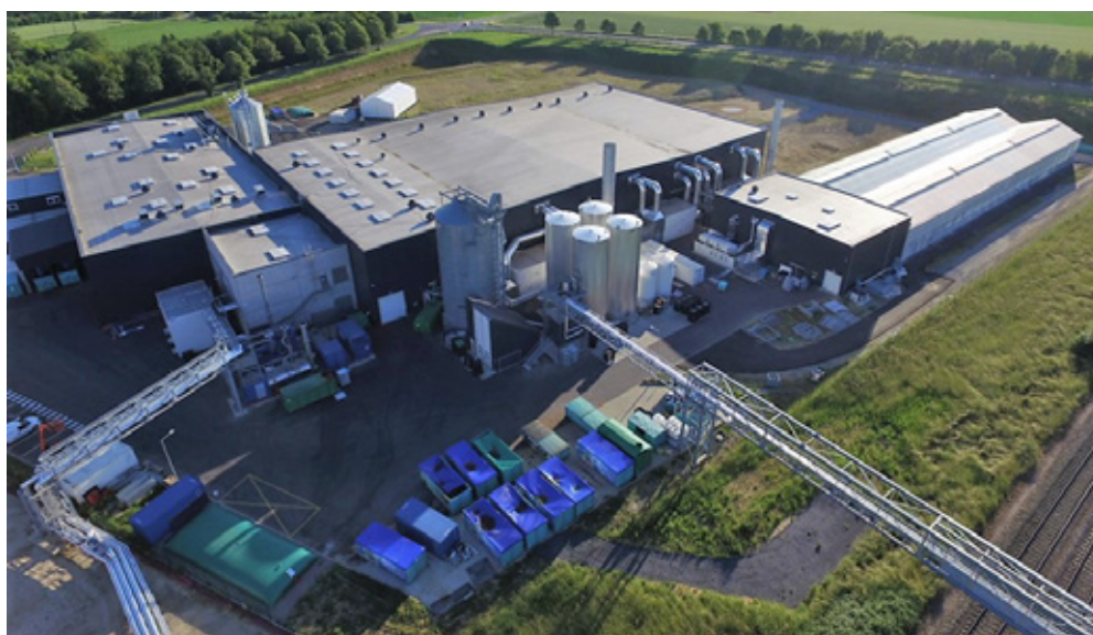
View of the farm in Nesle with four sectors; from right, anticlockwise, Reproduction, Growth, Sieving and Processing. Two separate piping brings in energy and agriculture feedstock.
