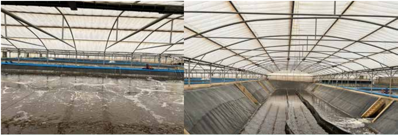
Grow-out ponds (left) and right, the treatments ponds with barriers to slow water flow and settle solids. Tilapia is stocked to control larvae of midge flies which are present in the organic matter in the digester.
