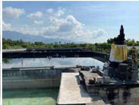
Ponds at UD Putra Gunung Sari Bahari during pond preparation for the next crop. Left, cement ponds and (right) ponds lined with 0.5mm HDPE liners.
