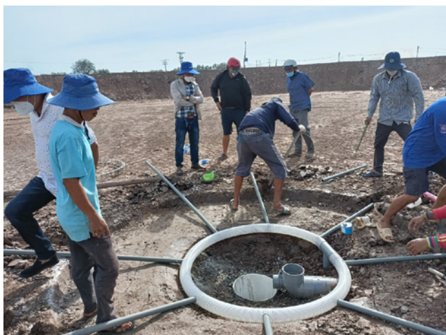
Construction of a central drainage system for a farm.
