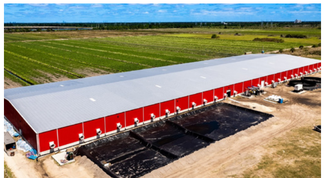
External view of the newly dedicated shrimp grow-out facility at Homegrown Shrimp USA.
