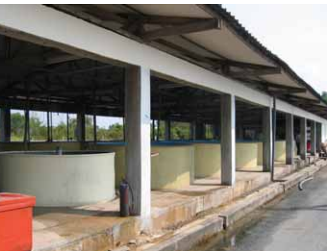
This part of the hatchery has 20 tanks, each with a capacity of 5 tonnes. A closed recirculation system is used to provide a better control of water quality and parameters.
