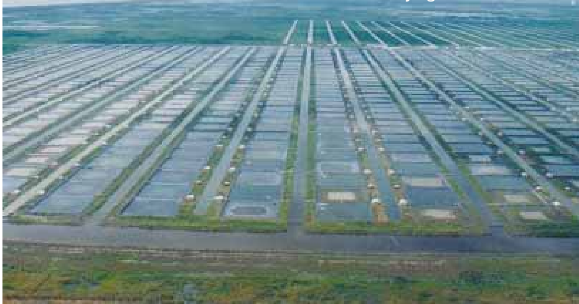
Plastic liners are extensively used in shrimp farms like the P.T. Dipasena project located in South Sumatra, Indonesia.
