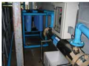
Water is cleaned by a series of filters
