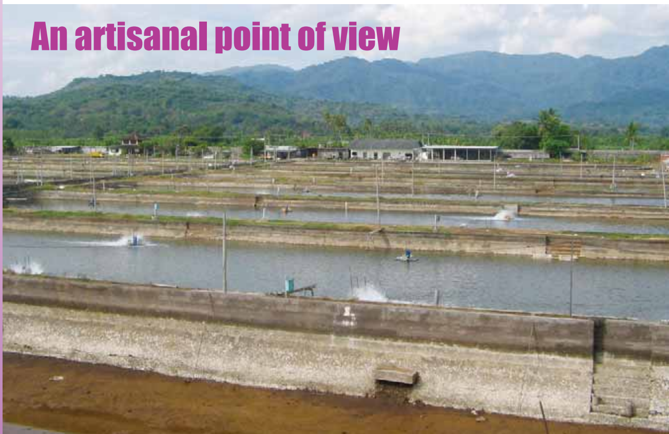
Wira has opted for rectangular shape ponds with cement dykes and clay soil bottom
