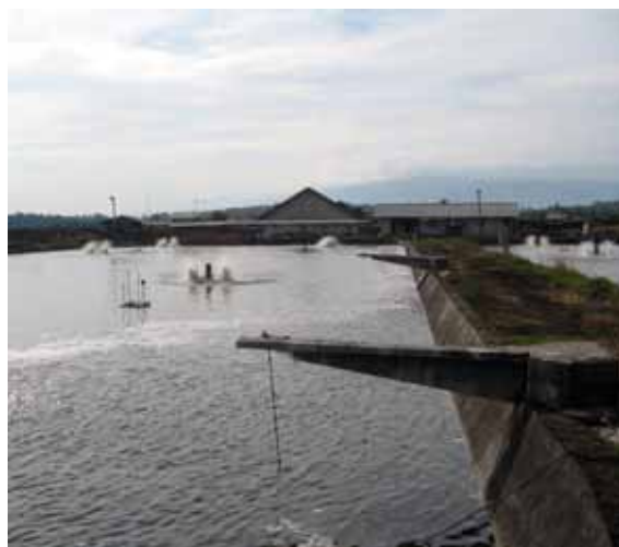
These are the cement platforms jutting into the ponds for regular sampling work. Note that there is no foundation pole in the pond
