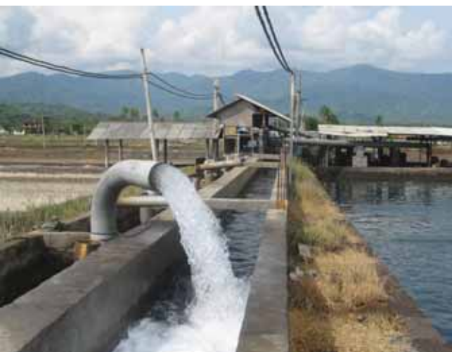
Pumping water from one and another reservoir ponds
