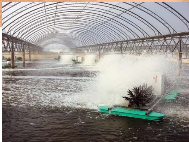
Inside view of ponds (Pictures courtesy of CPF).
