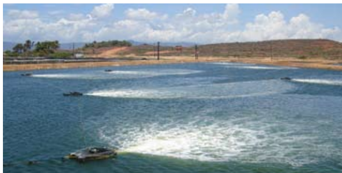
Pond with Aire-O 2 aerators shows the strong horizontal mixing.
