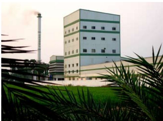
Growel Feeds Ltd, with a 10 tph Muyang extruder.
