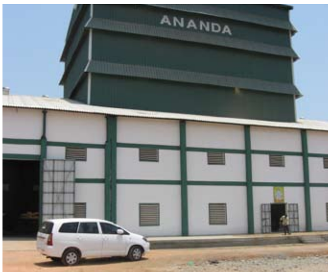
Ananda feeds with a 5 tph Muyang extruder.
