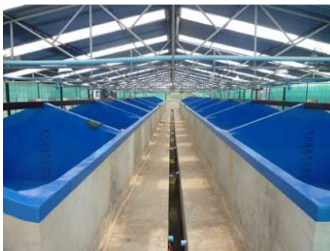
The hatchery is GAP certified by the Department of Fisheries. Inside of the hatchery, in between production cycles.
