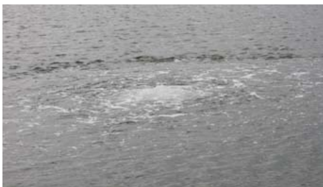
Fine bubbles from the diffused aeration system
