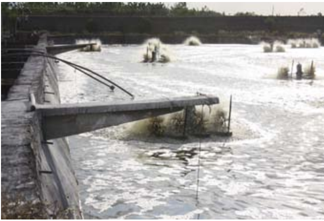
Concrete ponds with sampling platforms at Wira's farm
