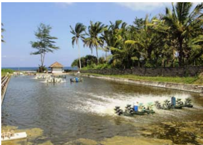
Pond where aerators push sludge to one end
