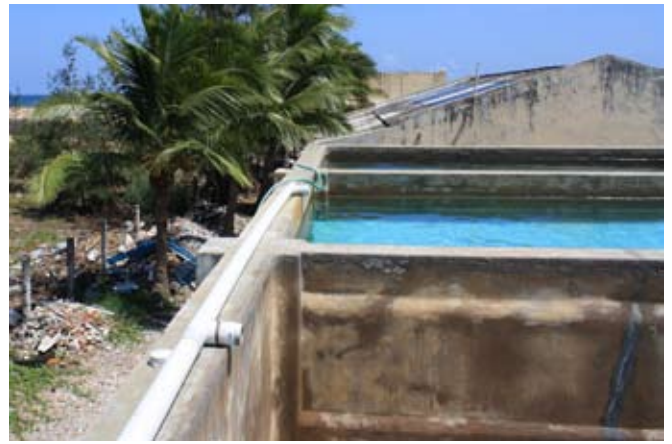
Seawater passes through a sand filter before storage in these treatment and reservoir tanks.
