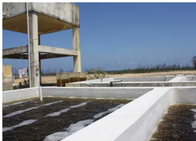
These are one tonne to 10 tonnes tanks for outdoor culture of live feeds
