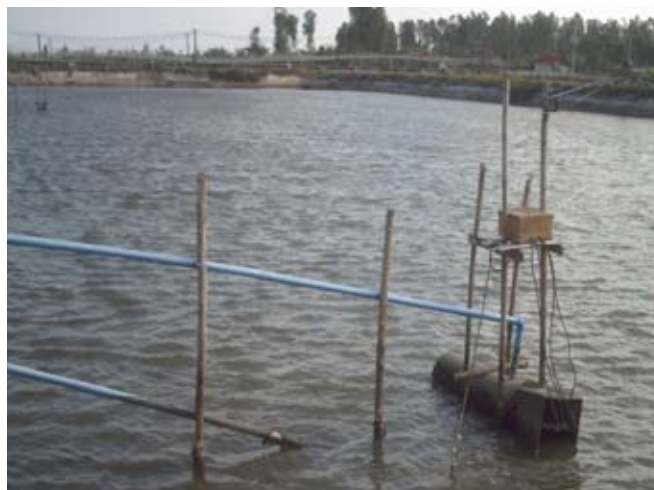
Treatment pond equipped with electrolysis machines.
