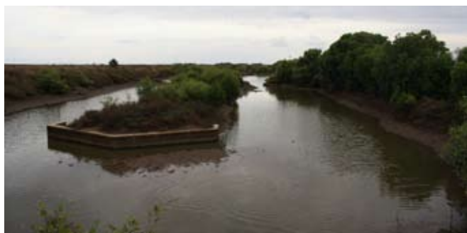
In this effluent treatment pond, mangroves trap sediments.
