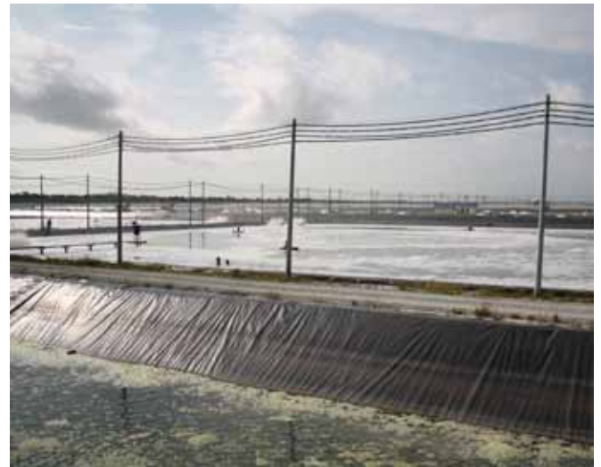
Overview of ponds and supply canal in phase 1
