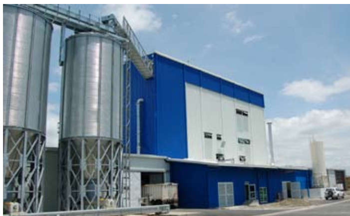
The new plant in Cañas, Costa Rica
