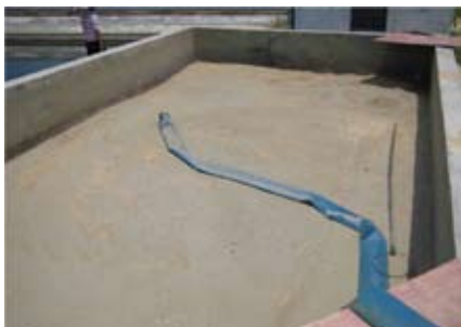
Cleaning the sand filter
