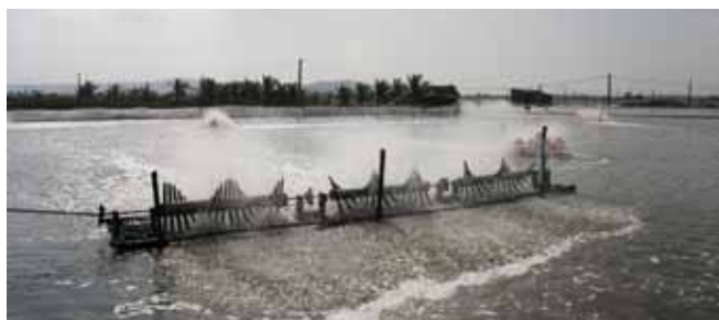
Spindle and paddle wheel aerators in operation
