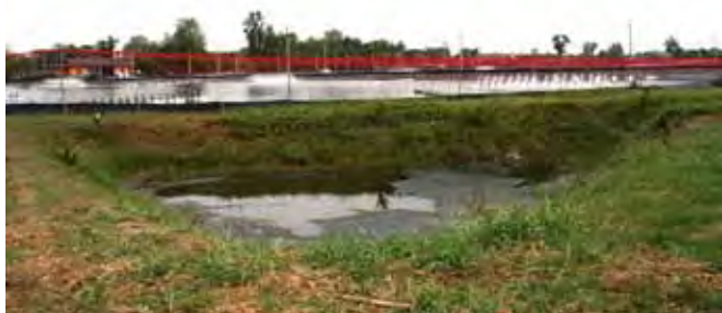
Sludge is removed to a settling pond next to the culture ponds
