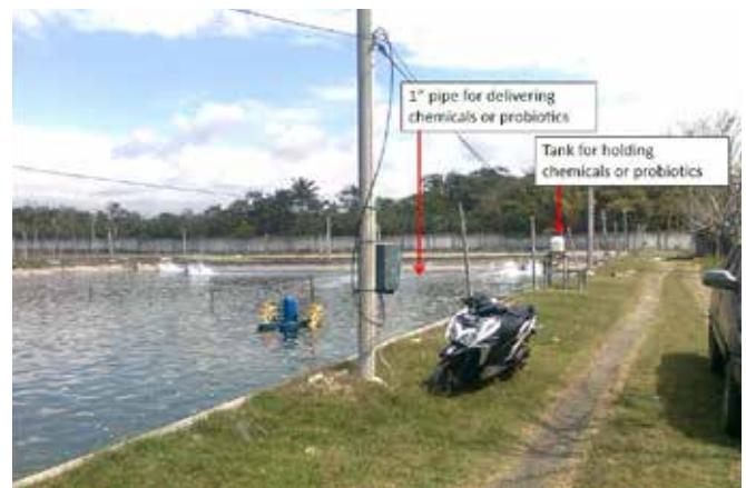
Delivery system for chemicals or probiotics directly to the sludge area.
