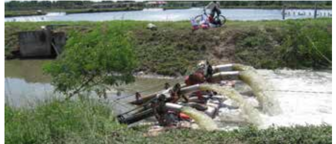
A makeshift dam made of bags of soil allows draining of the outlet canal to enable harvesting in low lying area.
