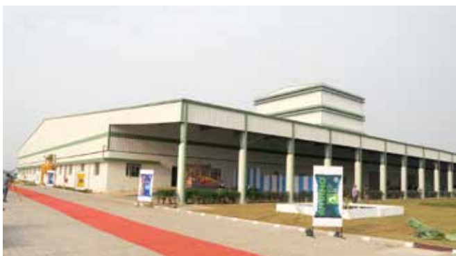
The new shrimp feed plant
