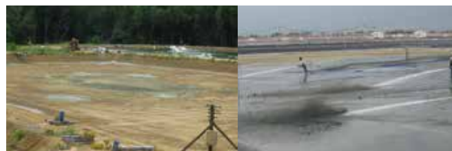
Figure 2. Ponds in Malaysia. Picture on the left shows a small mountain of sludge accumulated in the centre. Picture on the right, shows pond washing. Note the black sludge.
