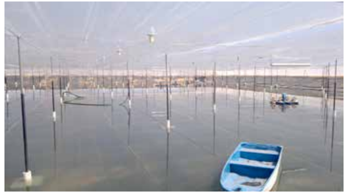
Rectangular tanks of 800 to 1000 tonnes in a greenhouse
