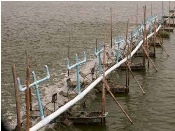
Saline water is channelled through a PVC pipe with many small holes placed in front of the aerator.
