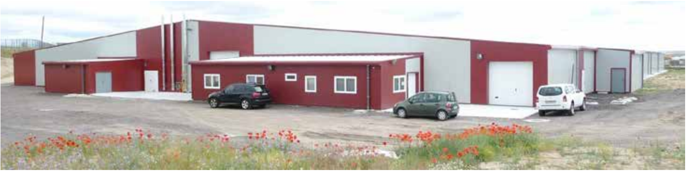
The Gamba Natural building. Inside there are 24 ponds
