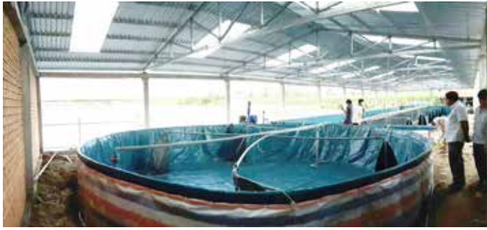
A new, 2-phase, shrimp nursery system currently under construction in Vietnam, with the technical support of Zeigler Bros. Inc. Credit: Ramir Lee.
