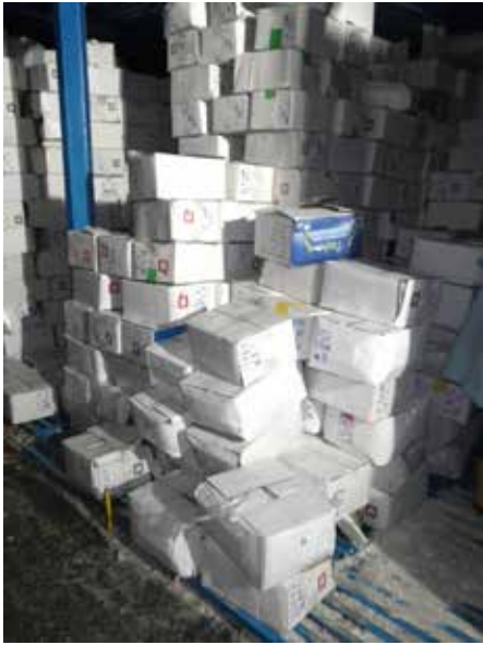
A bad example of an overloaded cold room
