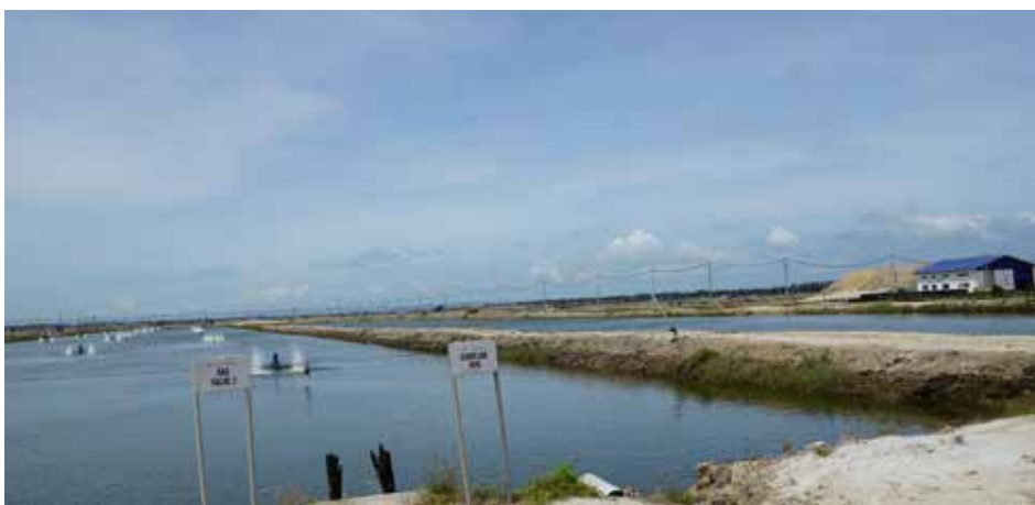
The IETS at iSharp, Phase 1. Aeration ponds with paddlewheels lead to the sedimentation pond. The marine outfall pump house is at the extreme right of the photo
