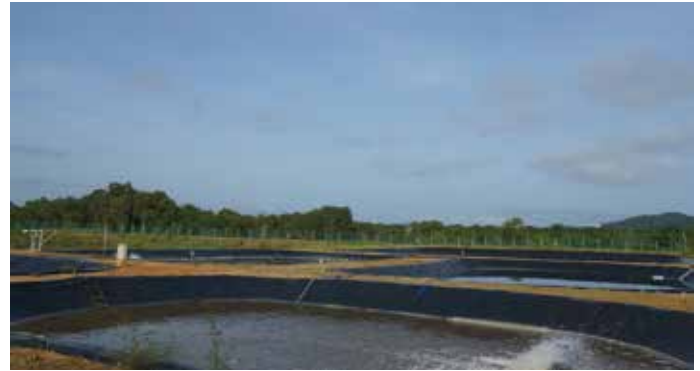
Aeration ponds at the hatchery
