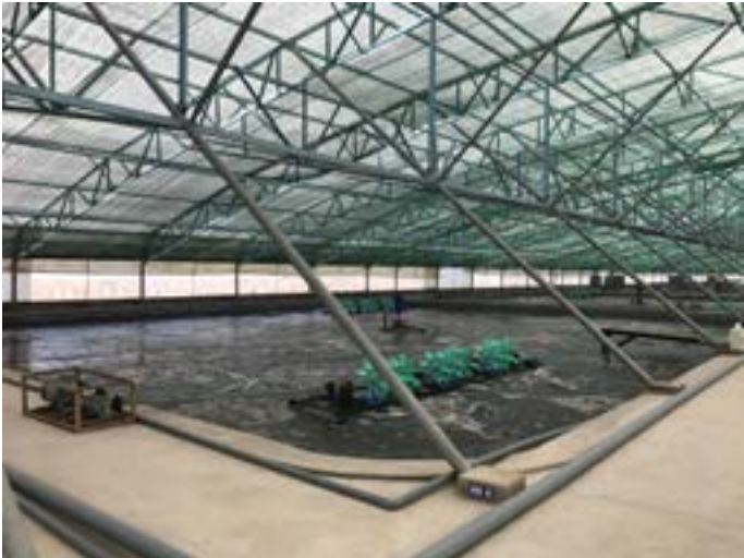
Paddle wheels in a grow-out greenhouse
