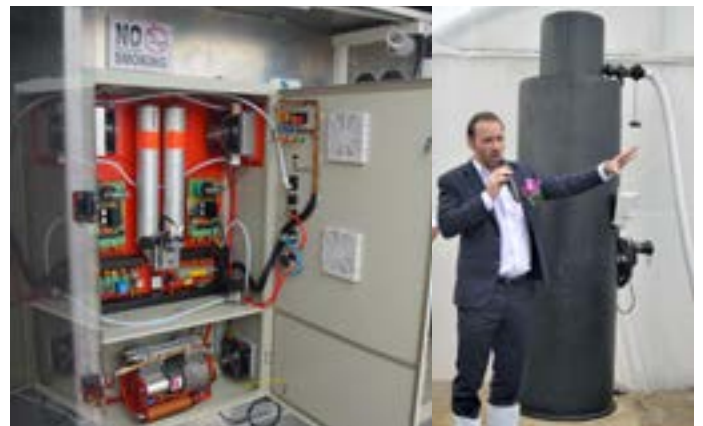
Thomas in front of the ozone tower. On the left is the mobile unit which generates ozone
