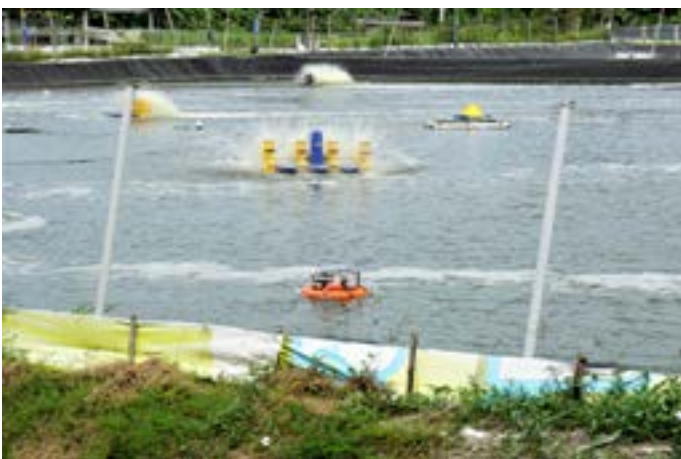
Lined pond with digital monitoring devices to continuously monitors temperature, pH, oxidation-reduction potential (ORP), dissolved oxygen and salinity.
