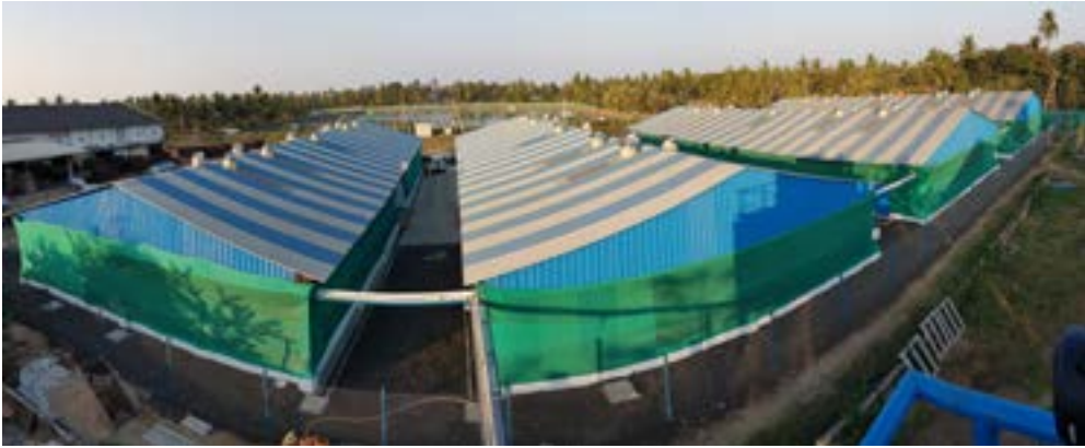
View of four units of the nursery with walls made of shading material. Photo credit: Anil Ghanekar
