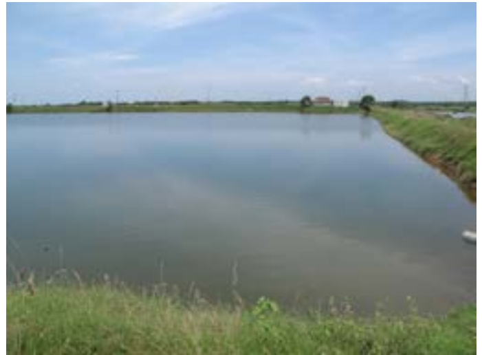
Intake water treatment pond in farm 2. For a sustainable business, this farmer treated the incoming water using a 2 ha reservoir.
