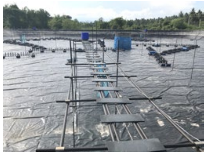
During the EMS crisis, many ponds were fully lined with polyethylene (PE) liners.
