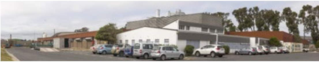
AgriProtein Technologies factory Philippi, Cape Town, the first commercial facility which grows BSF on a large scale and manufactures MagMeal, MagOil and frass. (Photo credit: AgriProtein)
