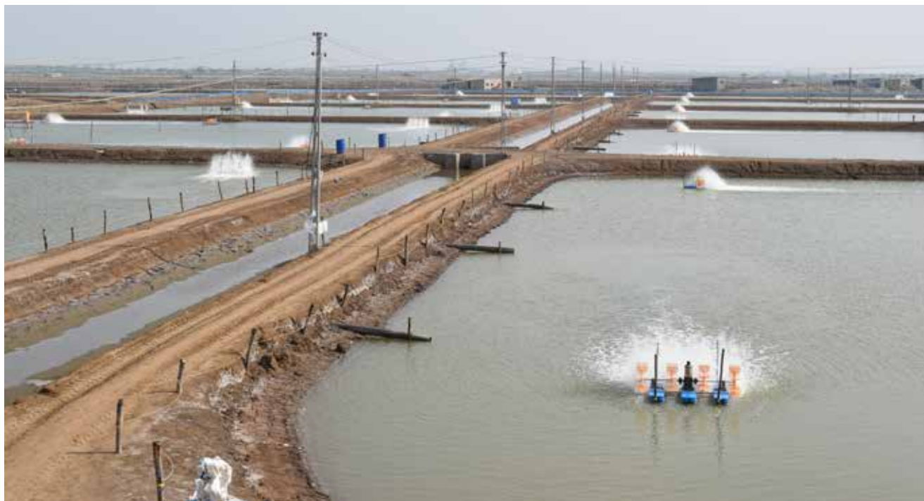
A new farm at Mayank Aquaculture, well designed with 40% of area for water treatment. Pond sizes are 0.5ha and water depth 1.8m. All ponds have a 4-step filtration system and a sludge removal system. There are separate ponds for sludge treatment and storage. All ponds have autofeeders to increase feed efficiency.
