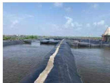
The different stages in water treatment include, from left, ponds for fast mixing of potassium permanganate and poly aluminium chloride, pipes to move water around for recirculation and right, ready to use water reservoirs.
