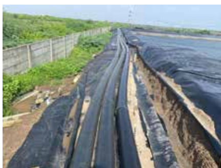
The different stages in water treatment include, from left, ponds for fast mixing of potassium permanganate and poly aluminium chloride, pipes to move water around for recirculation and right, ready to use water reservoirs.
