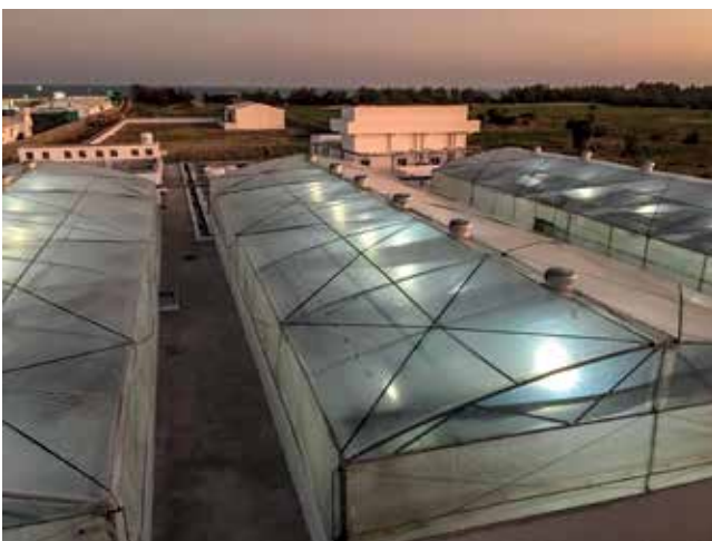
The new hatchery of Vaisakhi Bio-marine Pvt. Ltd in Pondicherry, India. There are more than 500 shrimp hatcheries in India which produced 70 billion post larvae in 2020.
