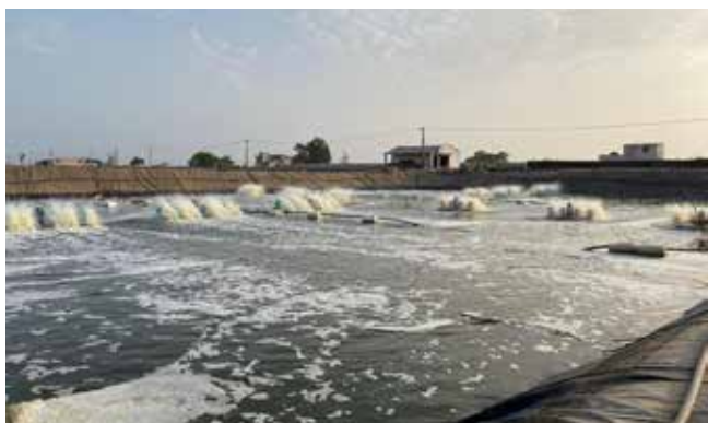
Grow-out pond with aeration devices – blowers and paddlewheels totalling 24HP.
