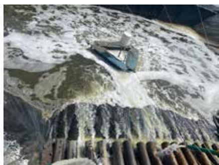
The different stages in water treatment include, from left, ponds for fast mixing of potassium permanganate and poly aluminium chloride, pipes to move water around for recirculation and right, ready to use water reservoirs.
