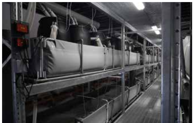
Sump tanks are all where most of the biological filtration happens before water is recirculated back to the grow-out tanks.
