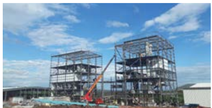
The Zambian factory under construction, May 2017 - © Aller Aqua Group A/S
