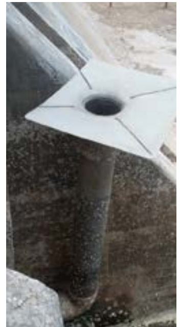
Drain pipe with the PVC sheet to divert shrimp away from the drain pipe.
