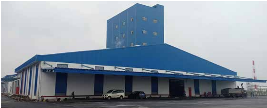
The 50,000 tpy shrimp feed plant in Thervoykandigai, Thiruvallur district, Tamil Nadu, India
